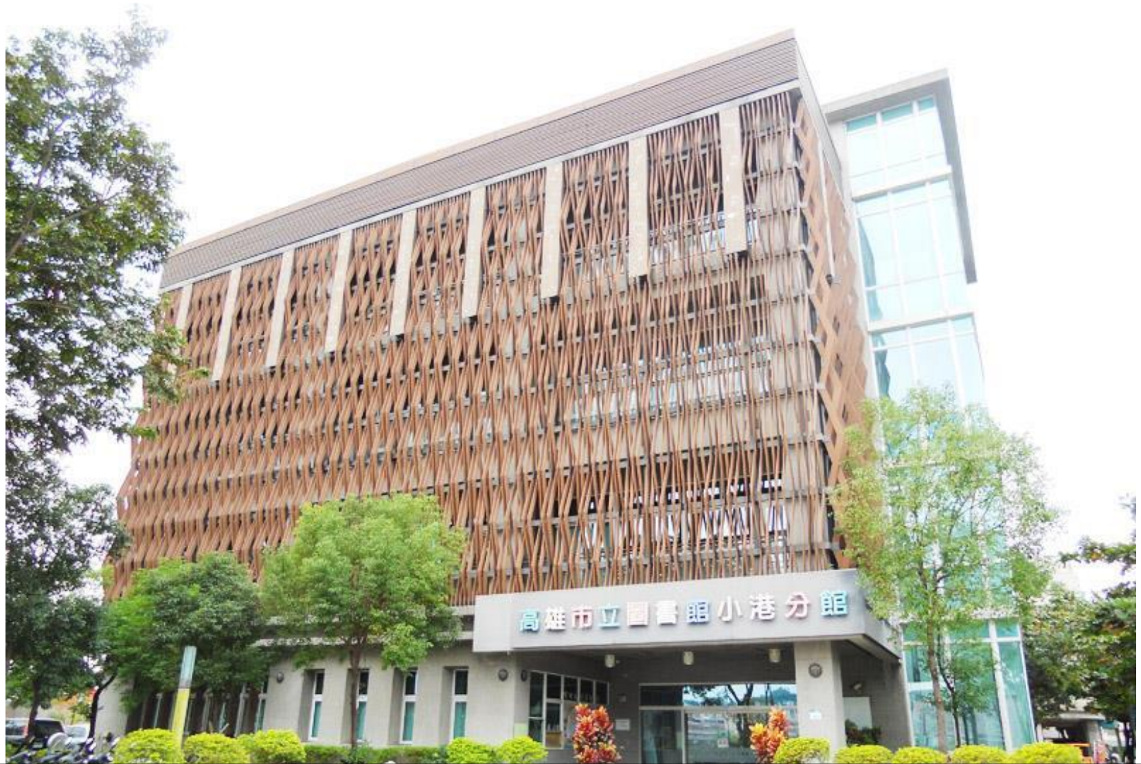
Kaohsiung Public Library Siaogang Branch.
